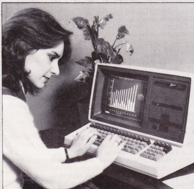
ZENITH DISKS — Zenith has added hard disk options to its Z100 range of business micros. Pictured is the 'all-in-one' ZW120, with 10Mb Winchester and 320K floppy. There's also a 'low profile' ZW100 for use with a separate colour or green screen monitor. The new machines come with 192K user RAM plus the usual Z100 specs of 8085, 8088, $100 bus, CP/M, Z-DOS (MSDOS) and Z-Basic. Prices for the hard disk machines start from a competitive £3,925. Zenith is on Gloucester (0452) 29451.
